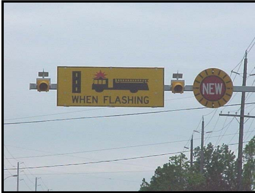
Figure 1 Typical Fire Hall Entrance Warning Sign
