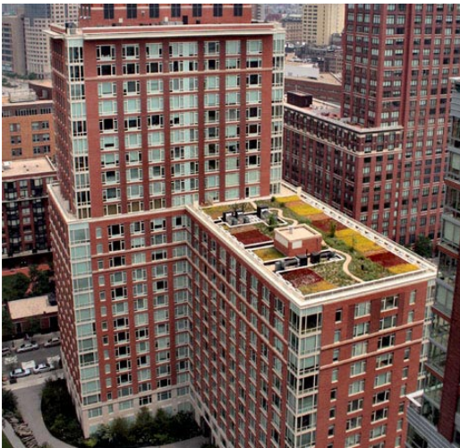
Green Roof Tribeca Green, New York City
