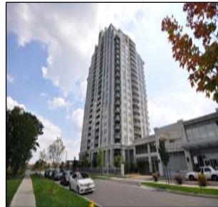
Condominium in Thornhill City Centre
