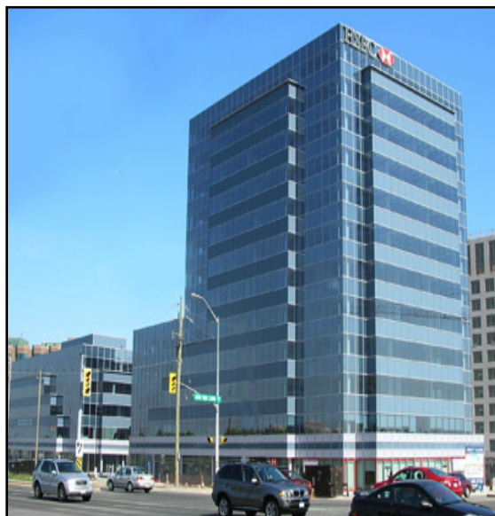
Liberty Square Markham – West Building Tallest office building in York Region to date – 12 storeys
