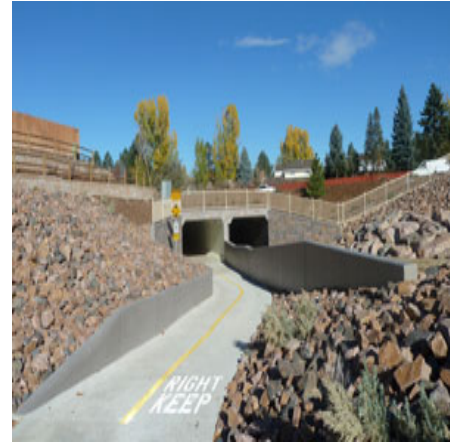
Figure 3 – Twinned Culvert/Pedestrian and Cyclist Crossing
