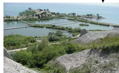
"End of Pipe" Controls
