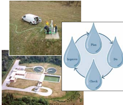
Keswick WPCP Upgrades
