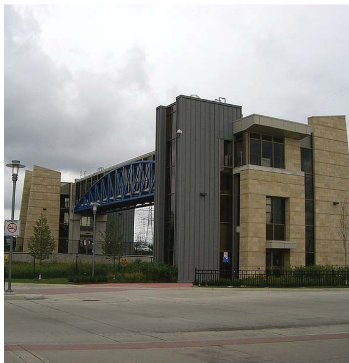
FIGURE 1.3A - PEDESTRIAN BRIDGE AT RICHMOND HILL CENTRE TERMINAL
