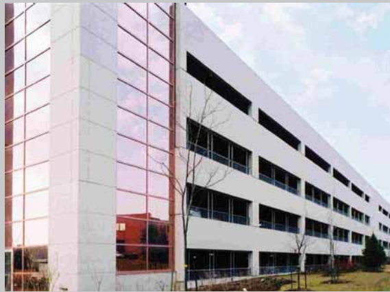
Markham Parking Structure built in phases
