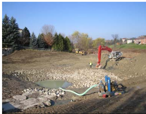
Shaping of Wetland Cells
