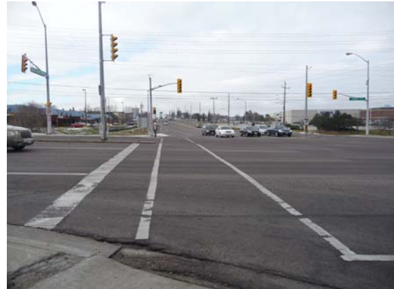
Without Zebra Crosswalk Markings
