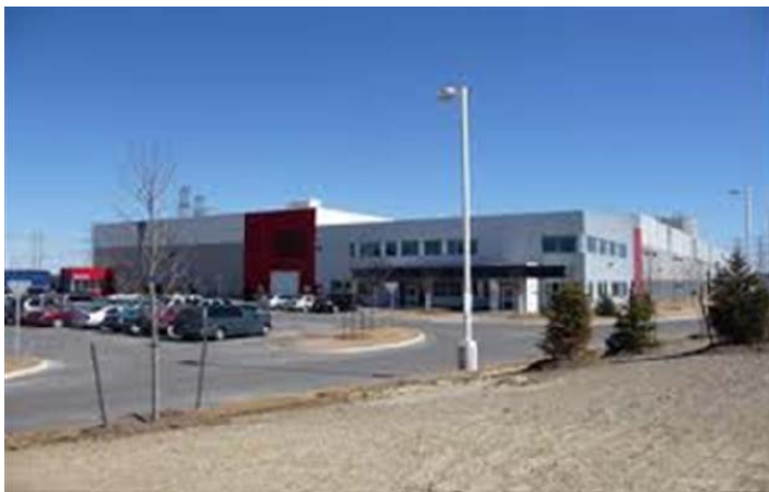
Dongara Pelletization Facility, Vaughan
