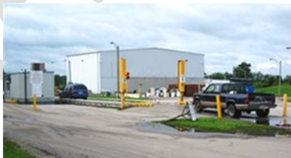
Georgina Transfer Station and Drop-off Depot, Georgina
