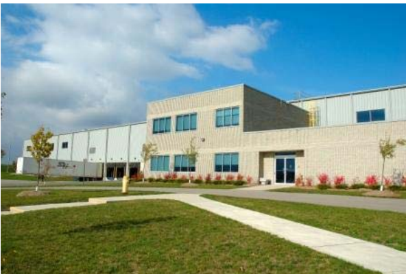
Waste Management Centre
