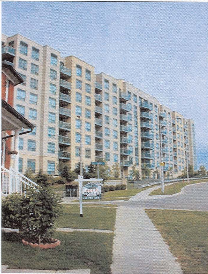
View – looking east along Bantry Avenue
