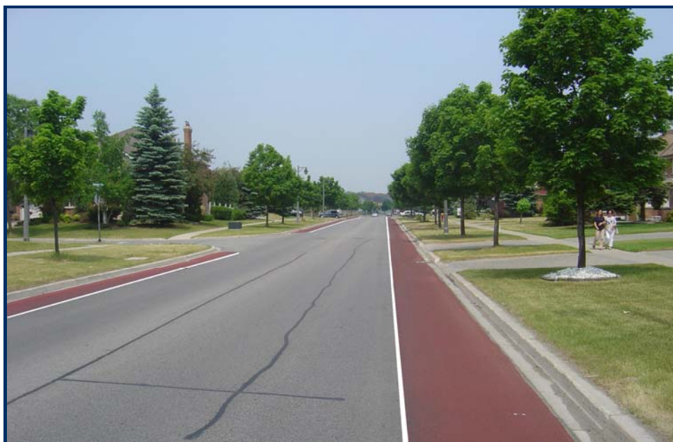
Figure 4.13 Microsurfacing – Town of Richmond Hill, ON
