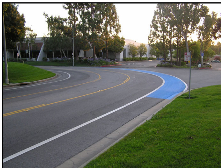
Figure 4.11 Coloured Pavement – Sunnyvale, California Source: Innovative Bicycle Treatments, ITE Web Seminar Presentation. Photo by John Brazil
