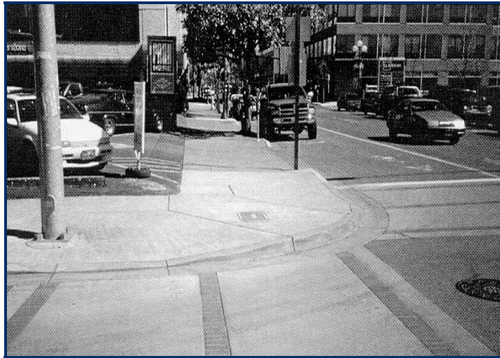
Figure 4.30 Reduced Curb Radius
