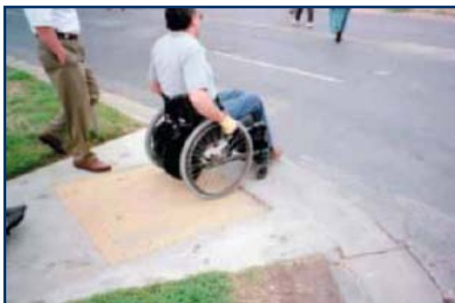
Figure 4.27 Typical Curb Ramp
