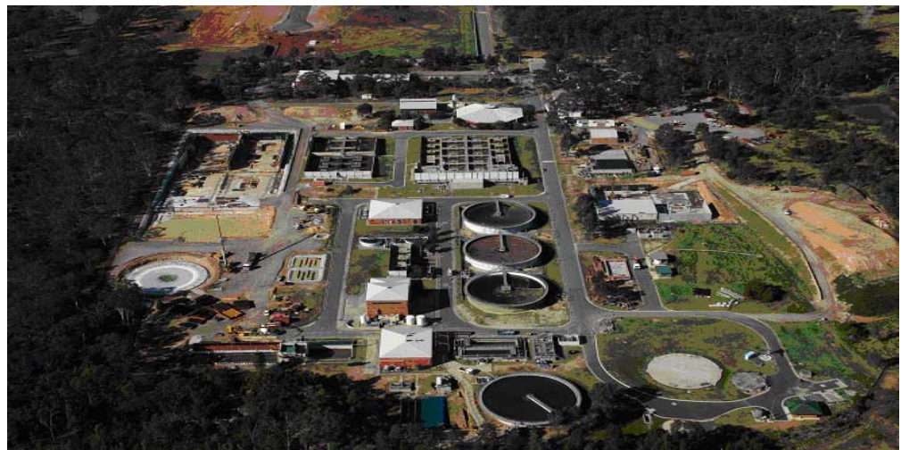
Rouse Hill Recycled Water Plant
