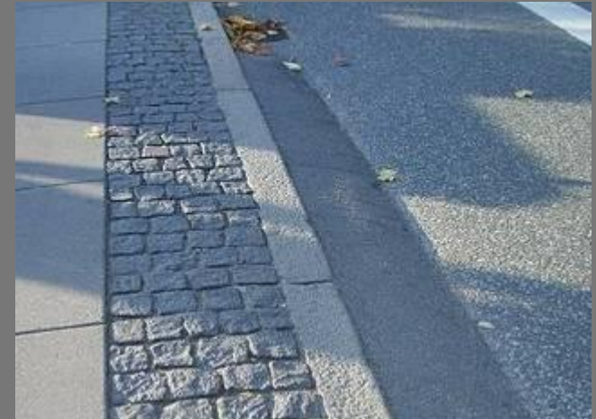
Mountable curb, Copenhagen
