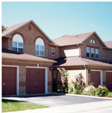
Springbrook Gardens Richmond Hill
