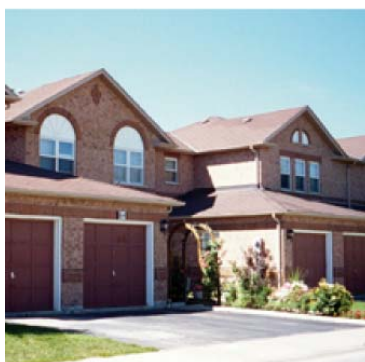
Springbrook Gardens Richmond Hill
