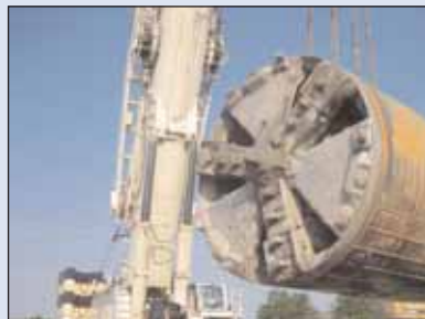
Removal of tunnel boring machine
