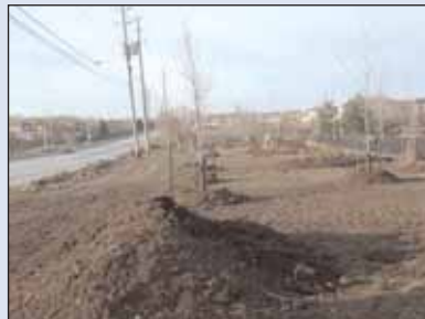
Restoration of Stone Mason compound (C-8)
