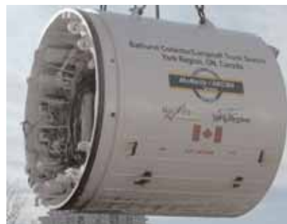
Lowering of EPBTM into C7 shaft.
