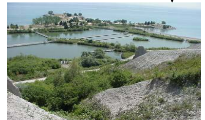
"End of Pipe" Controls
