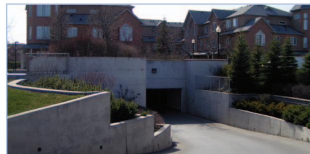
Underground parking, Markham Centre
