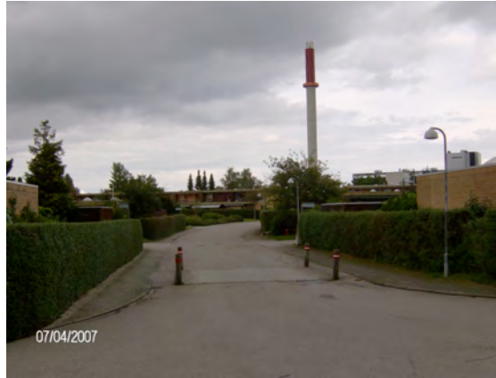
View from Residential Area
