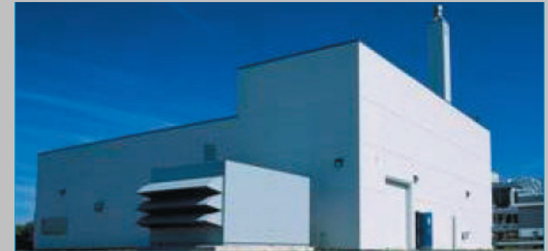
Markham District Energy Plant
