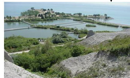
"End of Pipe" Controls
