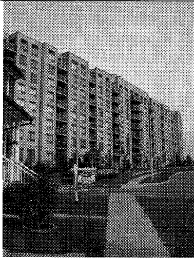
View – looking east along Bantry Avenue
