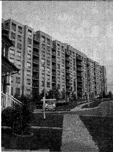
View – looking east along Bantry Avenue
