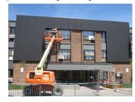
The building's heating system needs to draw air from the outside to refresh the air in the central hallway. Rather than drawing air directly from the outside and heating it, the system draws air from inside the metal panels of the sun-facing wall. On a cold winter day, the difference in temperature between the air inside the solar wall and the air outside can easily exceed 8° Celsius.
